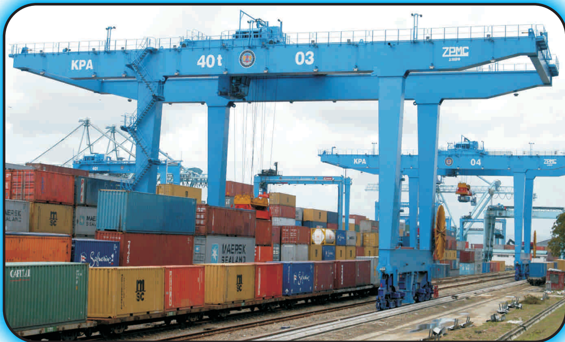
Rail mounted gantries at the terminal
